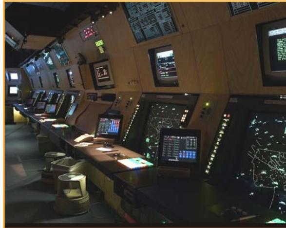
Tucson TRACON provides air traffic services around the clock (24/7), 365 days a year. U90 is classified as an ATC-8 facility, with five radar positions. STARS, the TRACON's newest system replaced ARTS IIIA in 2004. There are three control towers that operate in U90's airspace, Tucson ATCT, Davis-Monthan ATCT, and Ryan Field ATCT.
